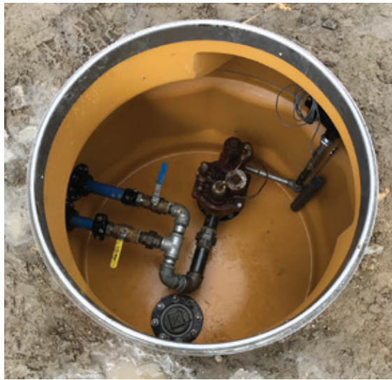
Before and after: Winter thaw and its corresponding runoff can be detrimental for secondary containment equipment at retail fueling sites (left). OPW's ElectroTite No-Drill Tank Sump (right) features factory installed sealed conduit ports, meaning it can be installed without pre-installation drilling, reducing the risk of water intrusion and unintended leak points.
