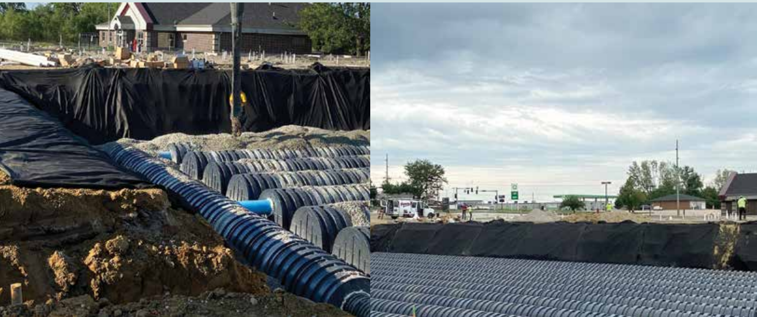
Whether used for retention, detention or infiltration, Xerxes stormwater engineers provide a site-specific engineered solution for each project based on system requirements, stormwater volume and site footprint.
