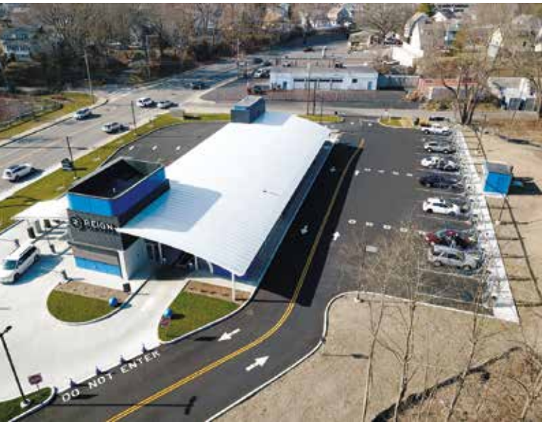
Clean lines, bold branding, and intuitive flow—this is a shining example of how a site can effortlessly guide customers from entry to shine while maximizing visibility on a main thoroughfare.
