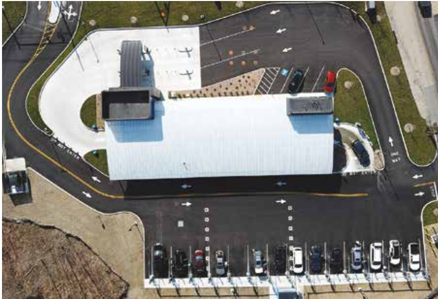
Separated and clearly marked entry/exit points, intuitive striping, and a natural traffic look keep cars moving smoothly while maximizing safety and throughput.
